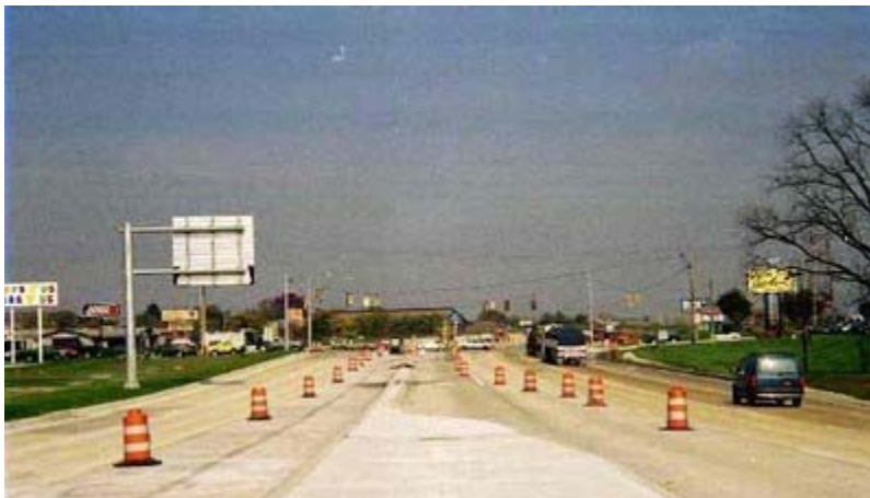
Median being completed near Kenneth Road. (PennDOT)
