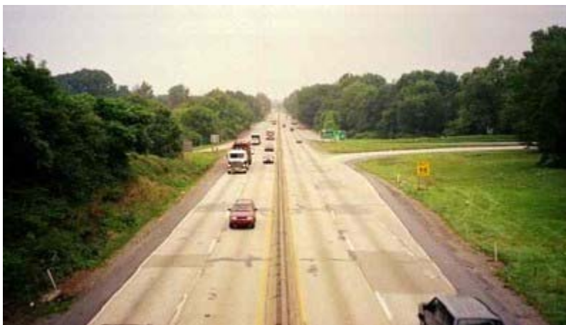
This was the section of US 30 west of New Holland Pike looks like it just came from the 1970s. (PennDOT)
