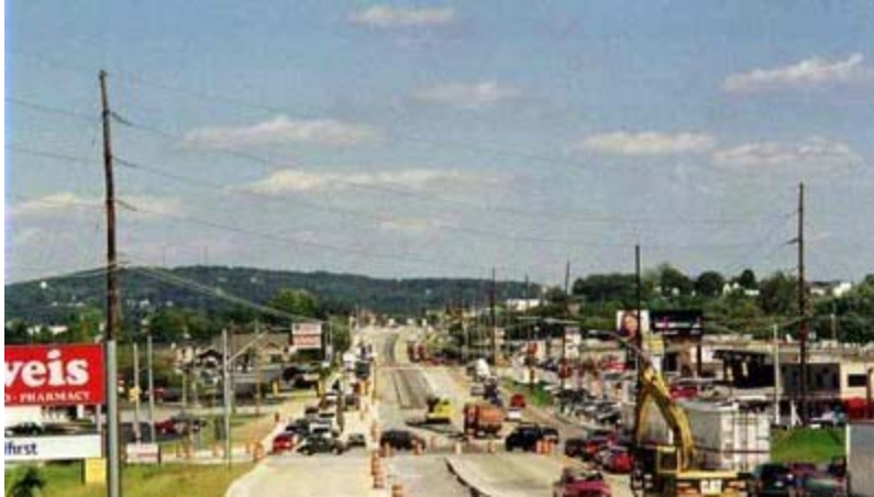
Work continuing between Pennsylvania and Roosevelt Avenues in York. (PennDOT)
