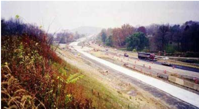
Construction occurring near Conestoga Creek. (PennDOT)
