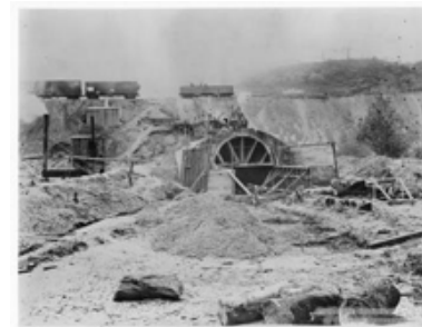
Tunnel entrance to steel mill under construction, ca. 1908
