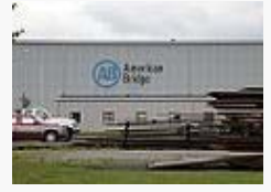
A building that is part of the American Bridge Company 's headquarters in Coraopolis.
