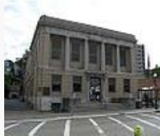
Coraopolis municipal building.
