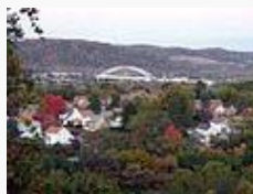
The Neville Island Bridge as viewed from a hill in Coraopolis.
