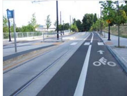
This bike lane has enough width for a bicyclist to comfortably ride between the curb and gutter and the adjacent travel lane.
